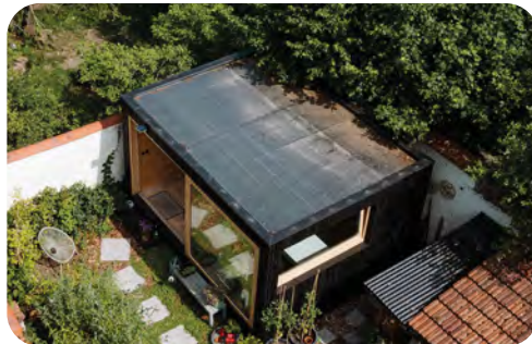
Dakbedekking in EPDM
